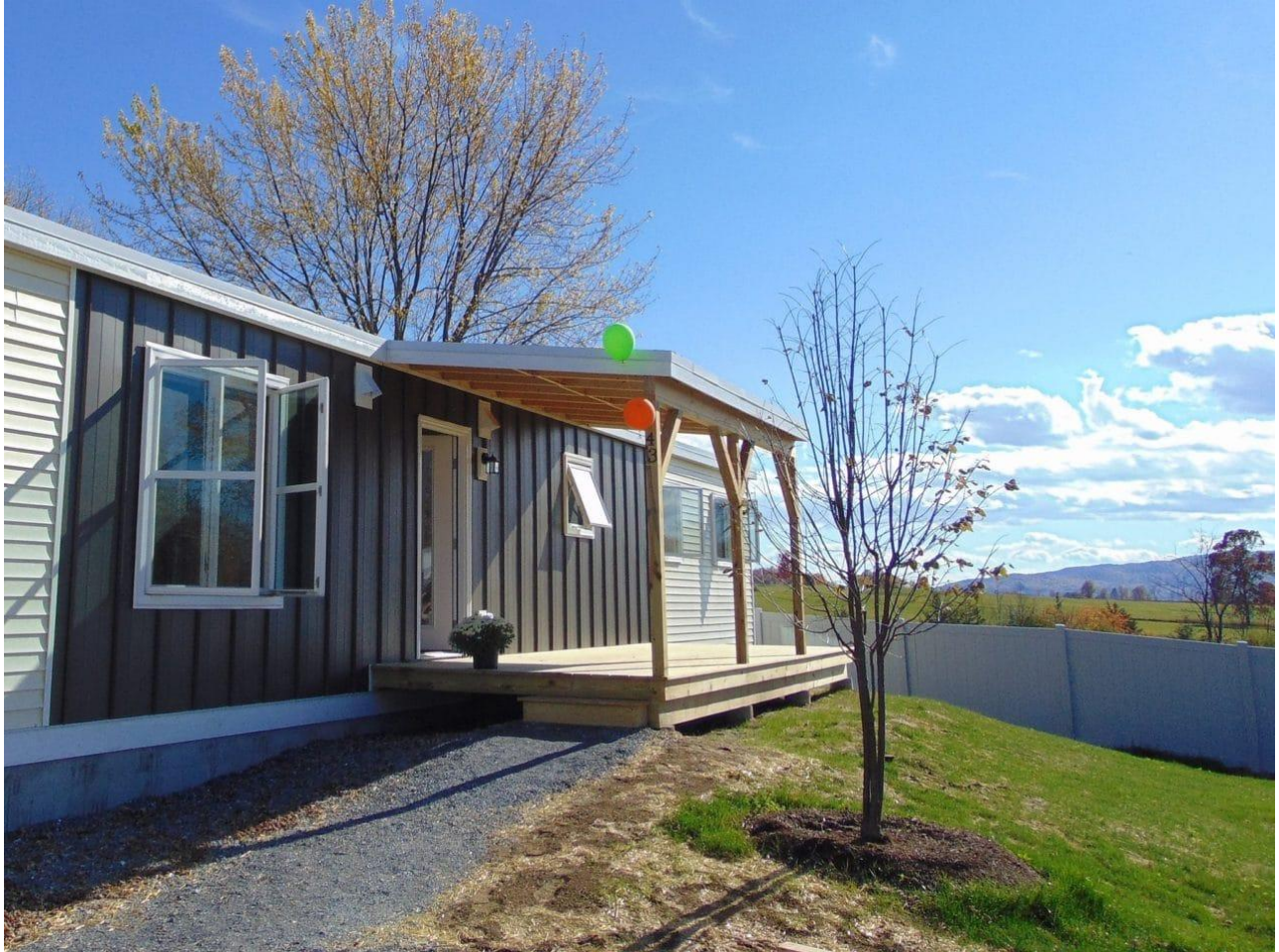
The McKnight Lane Redevelopment Project is located in rural Waltham, Vermont. Photo by Clean Energy Group.
