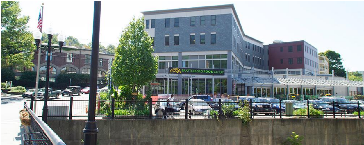
Co-op Plaza in Downtown Brattleboro , Vermont. Credit: Windham & Windsor Housing Trust
